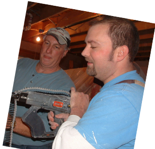
Tim and Micah use a borrowed drywall screw gun
