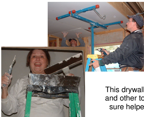
Tim and Micah use a borrowed drywall screw gun
